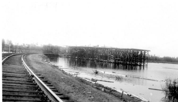
View looking east towards Longlac in 1941. An overhead (i.e., bridge) is under construction to pass over the Kenogami River and railway trestle to accommodate the new highway. Photo courtesy of Greenstone Historical Society.
